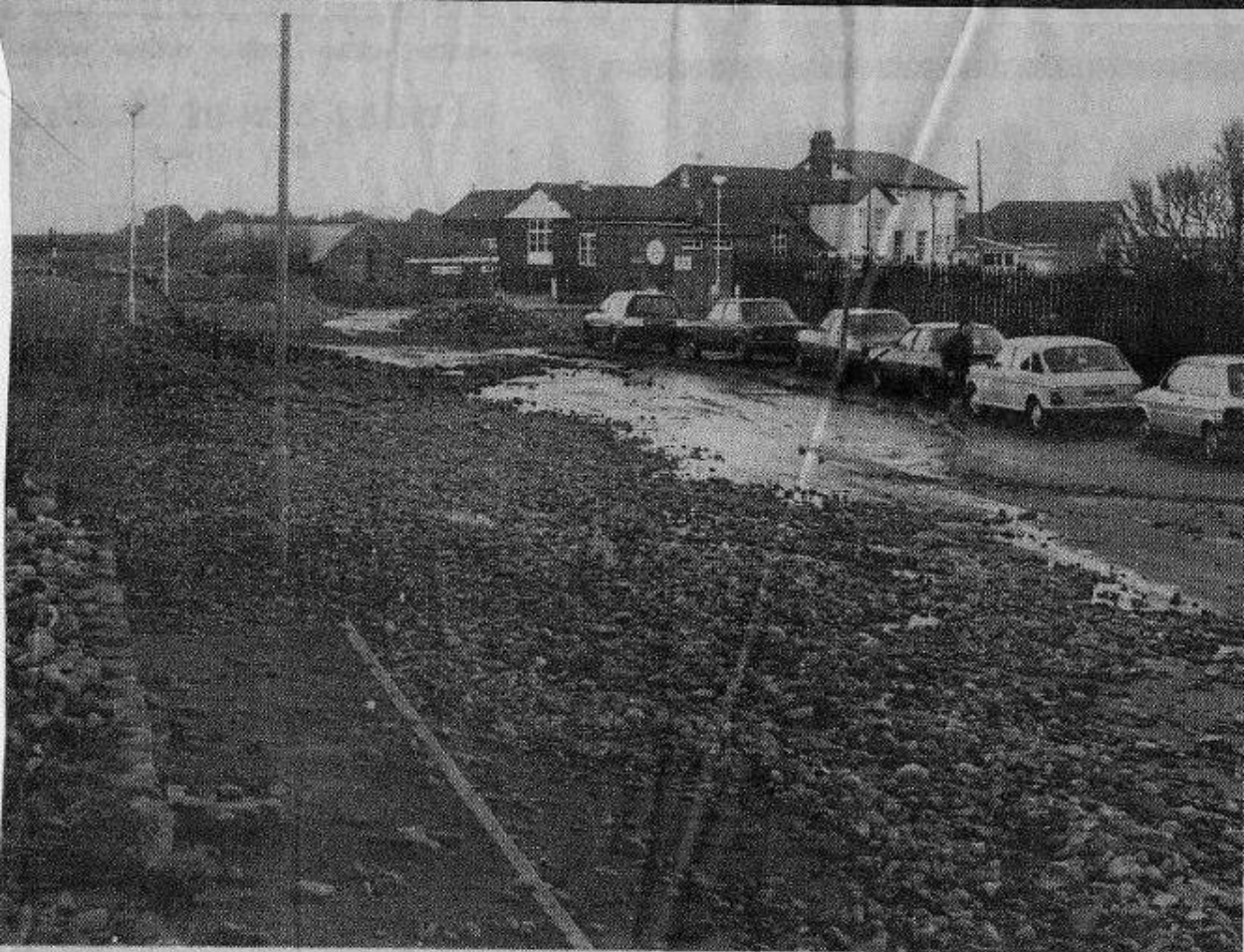
SHINGLE covers the road outside Minehead's Golf Club as the beach moved landwards.
